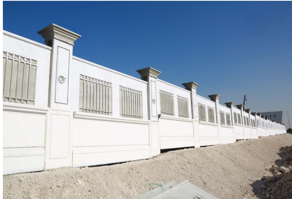
KAHRAMAA CENTRAL WORKSHOP
