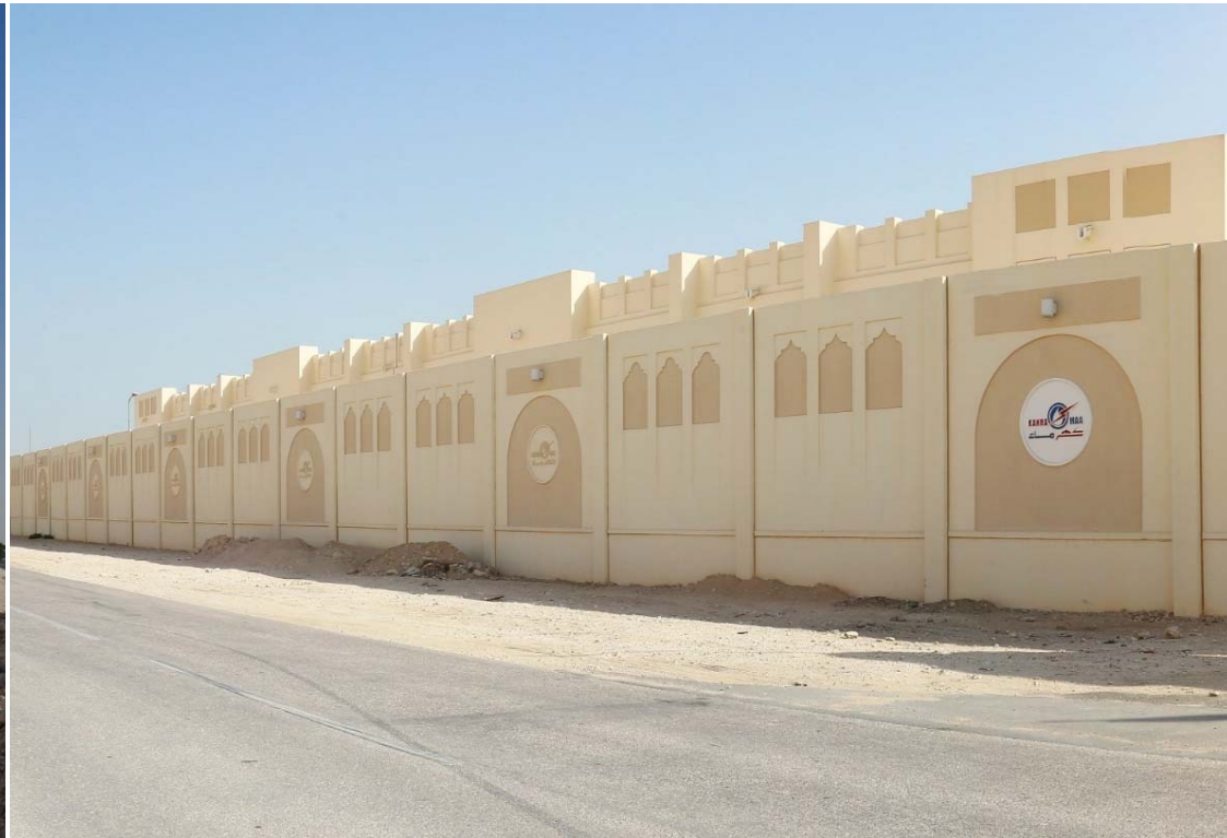
RESERVOIR PROJECT – DUHAIL
